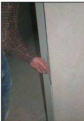
Figure 7: Installing a Foam Backer Rod
