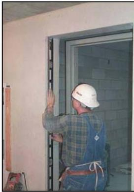
Figure 4: Drawing a Plumb Line
