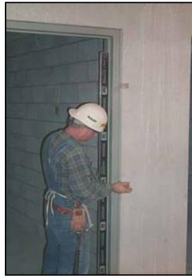
Figure 5: Inserting Wooden Shims
