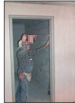
Figure 6: Drilling for Anchor Bolts
