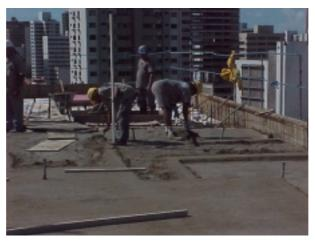
Figure 3: Floor screeding and setbacks for brick walls positioning
