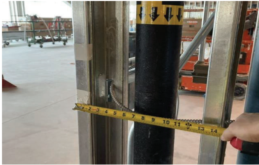
Figure 3: Photo Included in PDF Package Showing Pipe Location with Respect to Corner
