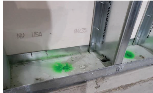
Figure 4: Fasteners Ready and Spray-Painted Green for Inspection
