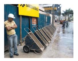
Picture 4 (a): Cleaned and positioned wheelbarrows in the sidewalk, waiting the concrete-mixer truck with the industrialized mortar.
