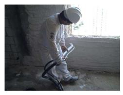
Picture 5 (a): Gypsum machine projector. Picture 5 (b): Plasterer projecting gypsum in the wall.
