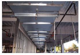
Figure 7: Flexible duct connection absorbs dimensional variation (Source: Iris D. Tommelein)
