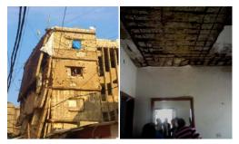
Figure 1-Damaged building, Spalling concrete
