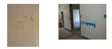
Figure 1: Left: information on the designed positions of the new structures. Right: work order sprayed on the wall.
