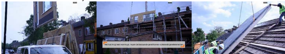
Figure 5: Installing prefabricated roof and façade elements (Sav, 2014).
