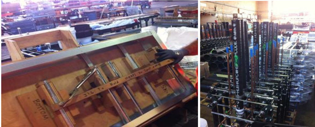
Figure 2 Welding jig on the left and stock of prefabricated modules on the right
