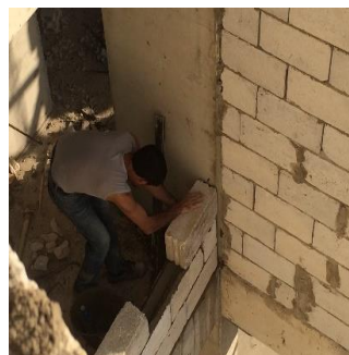
Figure 7: Working in awkward and restricted space
