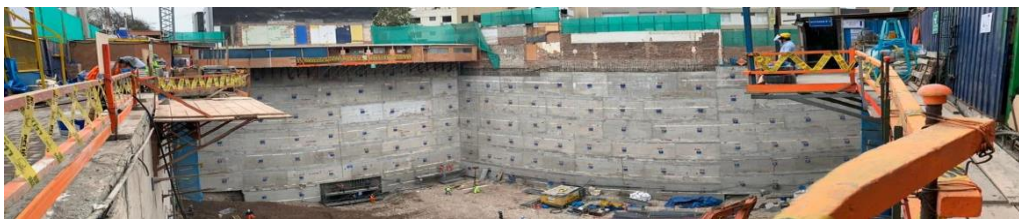
Figure 2. Panoramic view of the building of the anchored wall
