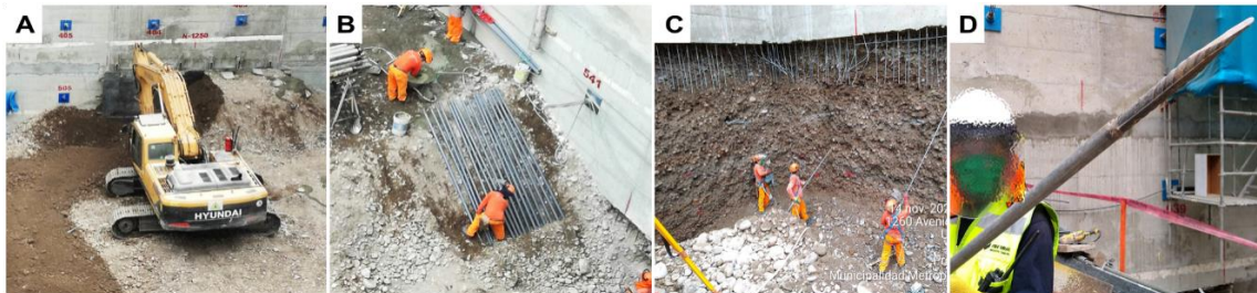
Figure 6. Improvements and innovations in basement construction.
