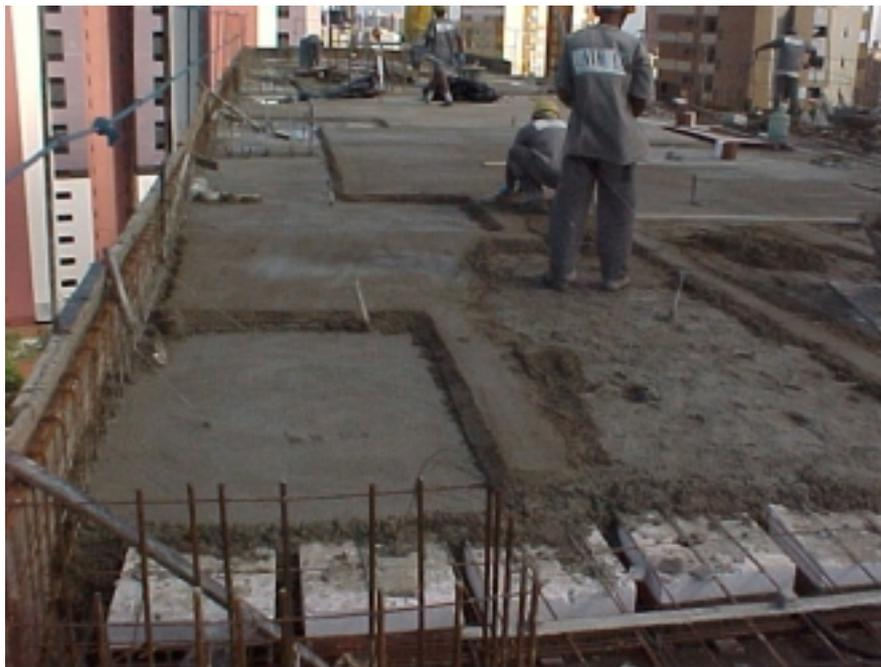
*Figure 4: Molding of slab with concrete mixed on site*
