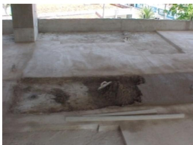
Figure 2: Floor screed executed with 50mm thickness
