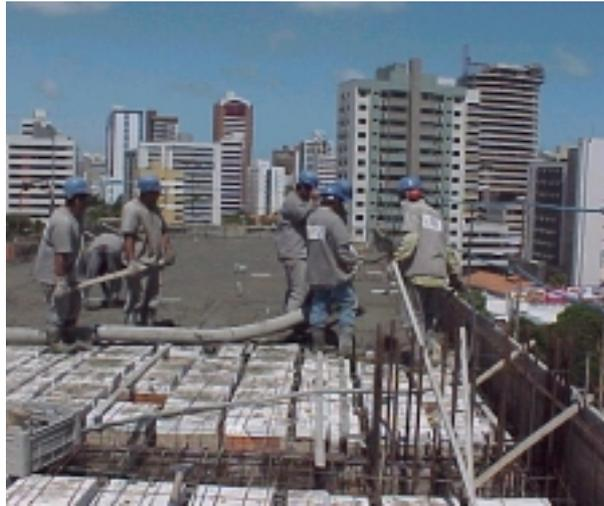
*Figure 2: Concrete pouring on the top of the ceramic and polystyrene blocks*
