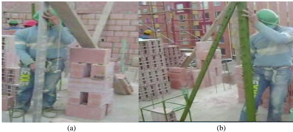
Figure 5: (a) Traditional Masonry Guiding device; (b) New Masonry Guiding Tool
