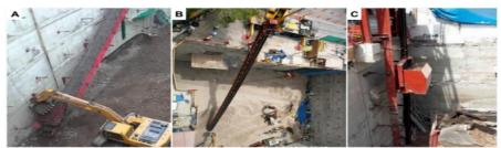
Figure 4: Alternatives to remove material for the seven, eight and nine basements.
