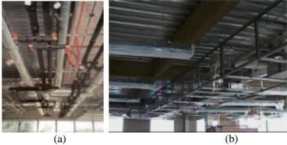
Figure 1: (a) Traditional horizontal distribution of building services (b) Installed prefabricated horizontal distribution units
