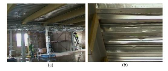
Figure 5: (a) Units being installed on site (b) damaged floor-pans causing installation problems
