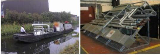
Figure 7: (a) Units being delivered to site via canal barge (b) Horizontal distribution units prior to installation
