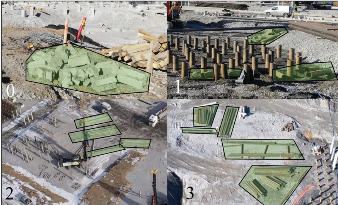
Figure 1: Four Examples of Observed Pile Waste Inventories
