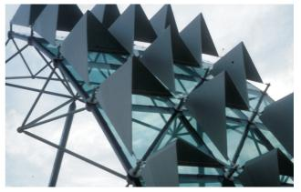
Figure 7: Mock up of aluminium sunshades and their fixing to the glazing system.
