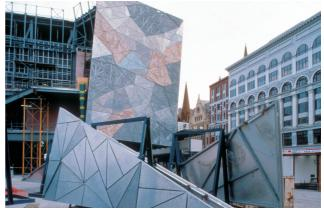
Figure 8: Apparent random fractal geometry based on a pinwheel used at Federation Square.
