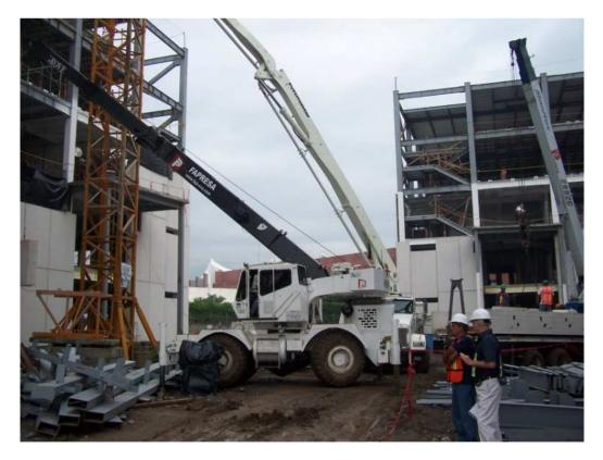
Figure 6: Installation of concrete facades with new sequence
