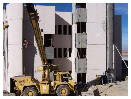
Figure 1: Installation of concrete facades in process (2008 project)
