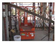
Figure 5: Material and Equipment Storage Confines due to Limited Floor Space in Workface Area
