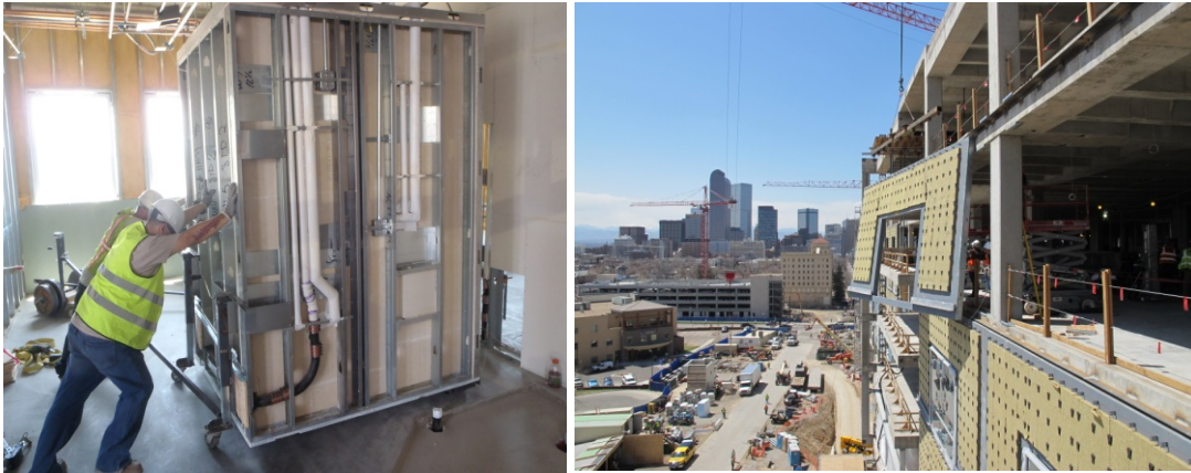
Figure 2: Typical Prefabricated Bathroom Pod & Wall Panel
